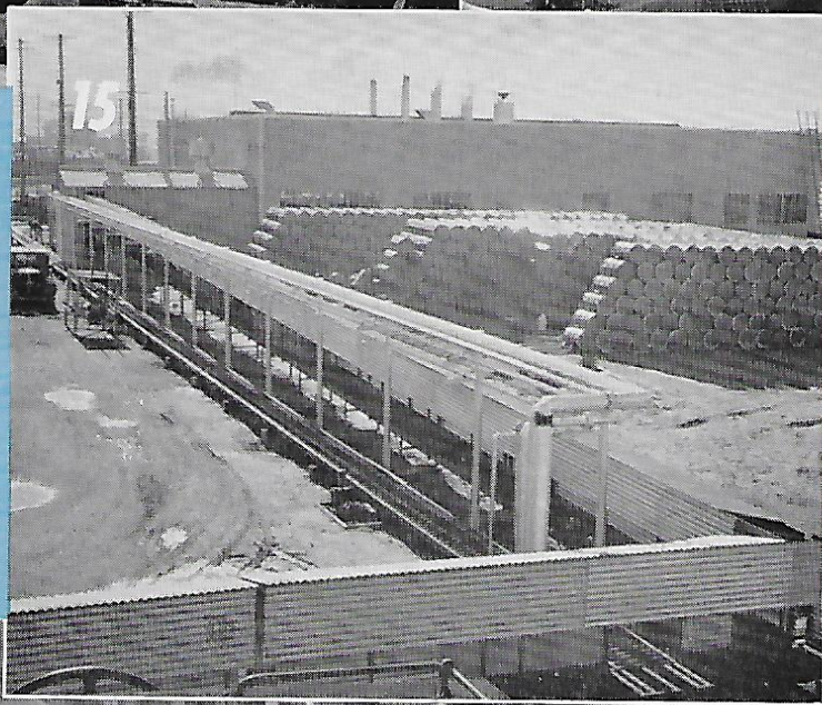
(15) Drums, just as good as new, now go via covered conveyor to one of several filling stations.
