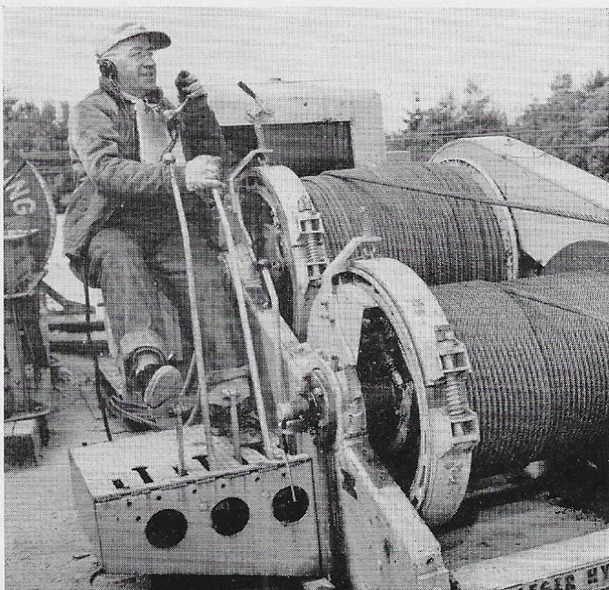
Equipment used in unreeling and spinning at the job site includes a telephone system and several "walkie-talkies", as the mile-long job requires coordination.
